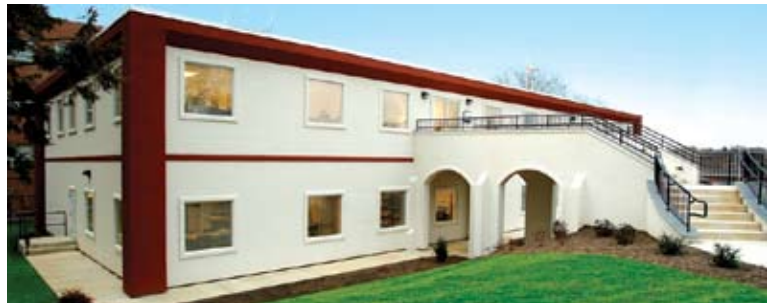
The facility is occupied and operational in less than five months.
